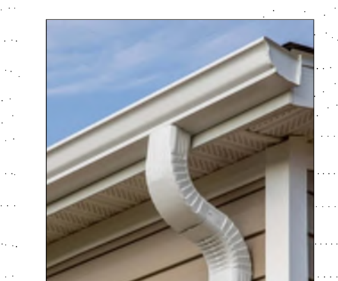
⑦ ALUMINUM GUTTERS & DOWNSPOUTS
