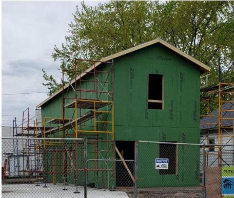
A Winona Habitat home under construction in 2021.
